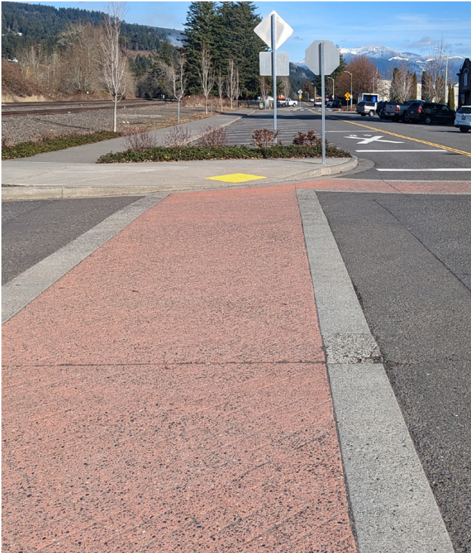
Existing crosswalk improvements for pedestrians.
